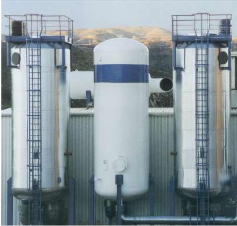
Figure 4—Example of an oxygen VSA
