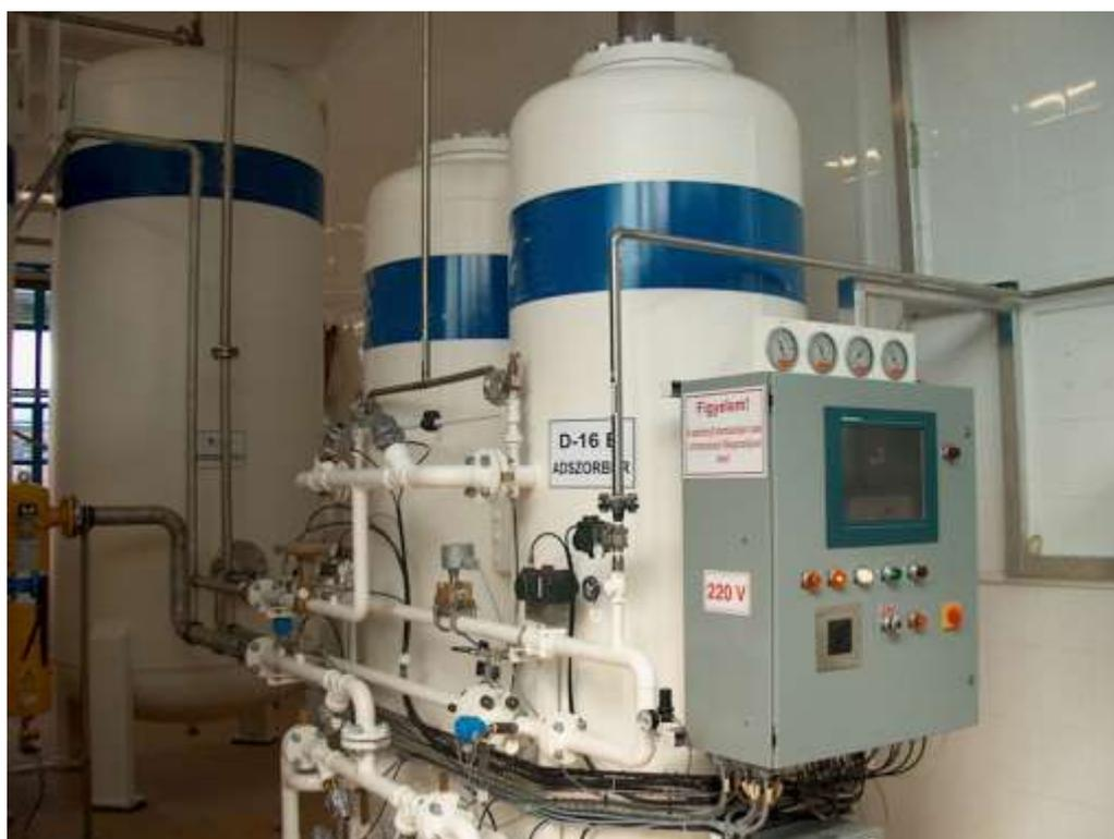
Figure 9—Example of a Nitrogen generator
