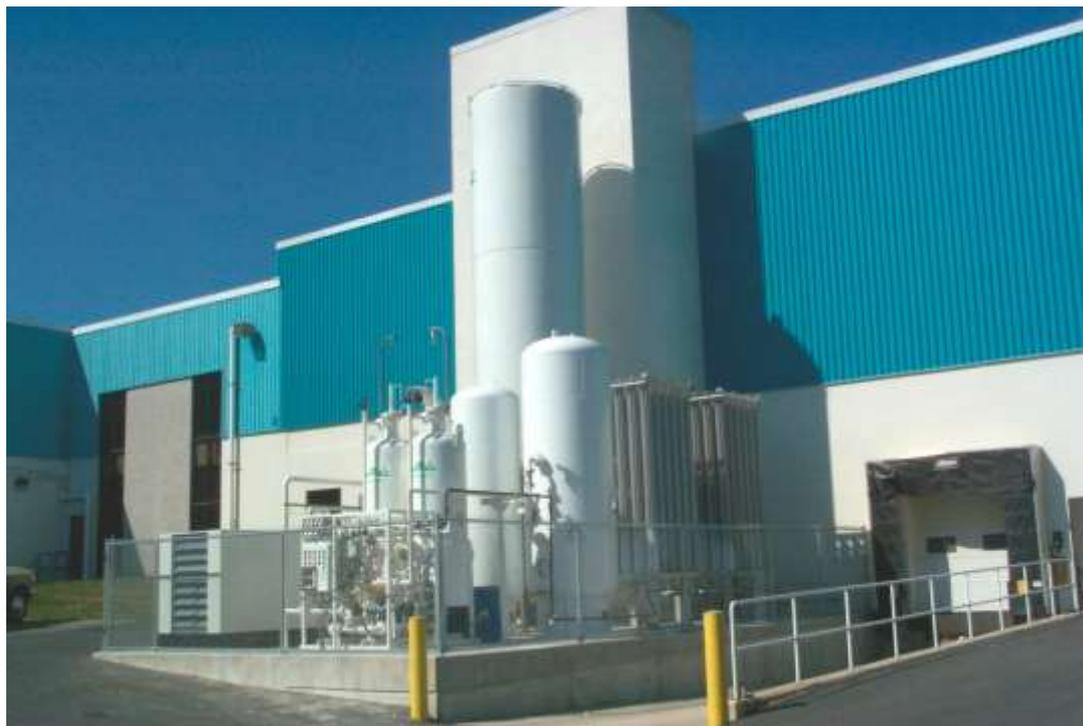
**Figure 10—Example of a nitrogen generator (Photo courtesy of Air Products and Chemicals)**
