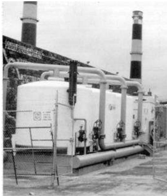
Figure 5—Example of a Three-bed oxygen PSA
