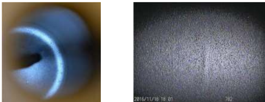
Figure 8 Internal views of cylinder K93.1
